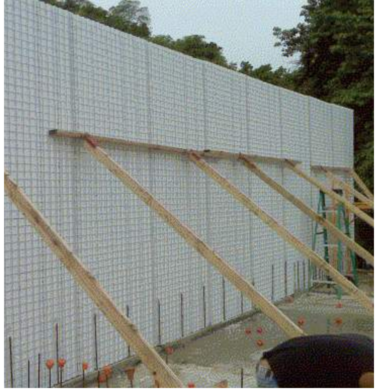
Photo 5: Temporary diagonal wall bracing.
