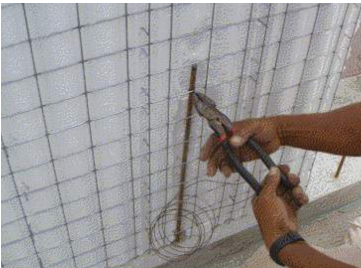
Photo 1: Connection of wire meshwork to foundation rebar anchorage using wire ties.
